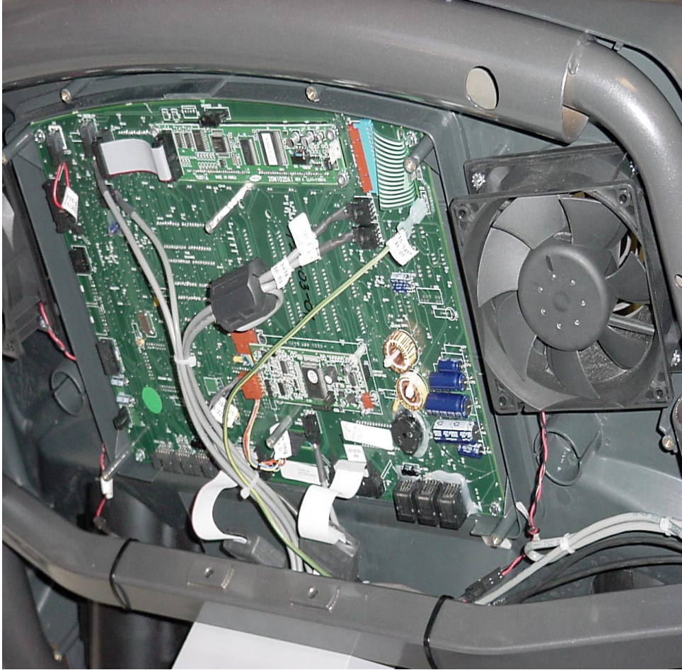
Complete wiring view of the back of a Pro Tread display
